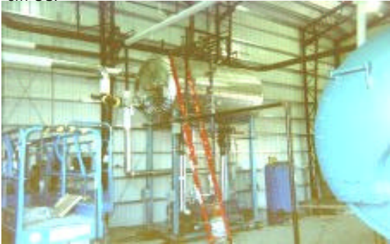
Above: Moss 100,000 lb./hr. spray deaerator at a large industrial textile company. Below: Moss 41,000 lb./hr. high pressure condensate return/deaerator system being installed at a large sawmill operation in the western US.
