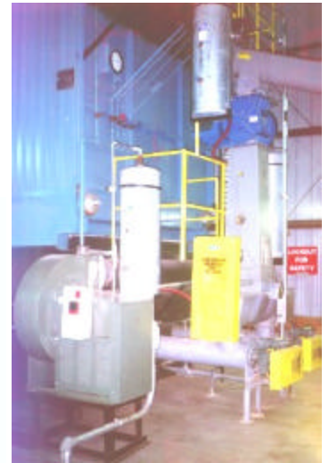
Moss watertube boiler installation with gasifier combustion system.
